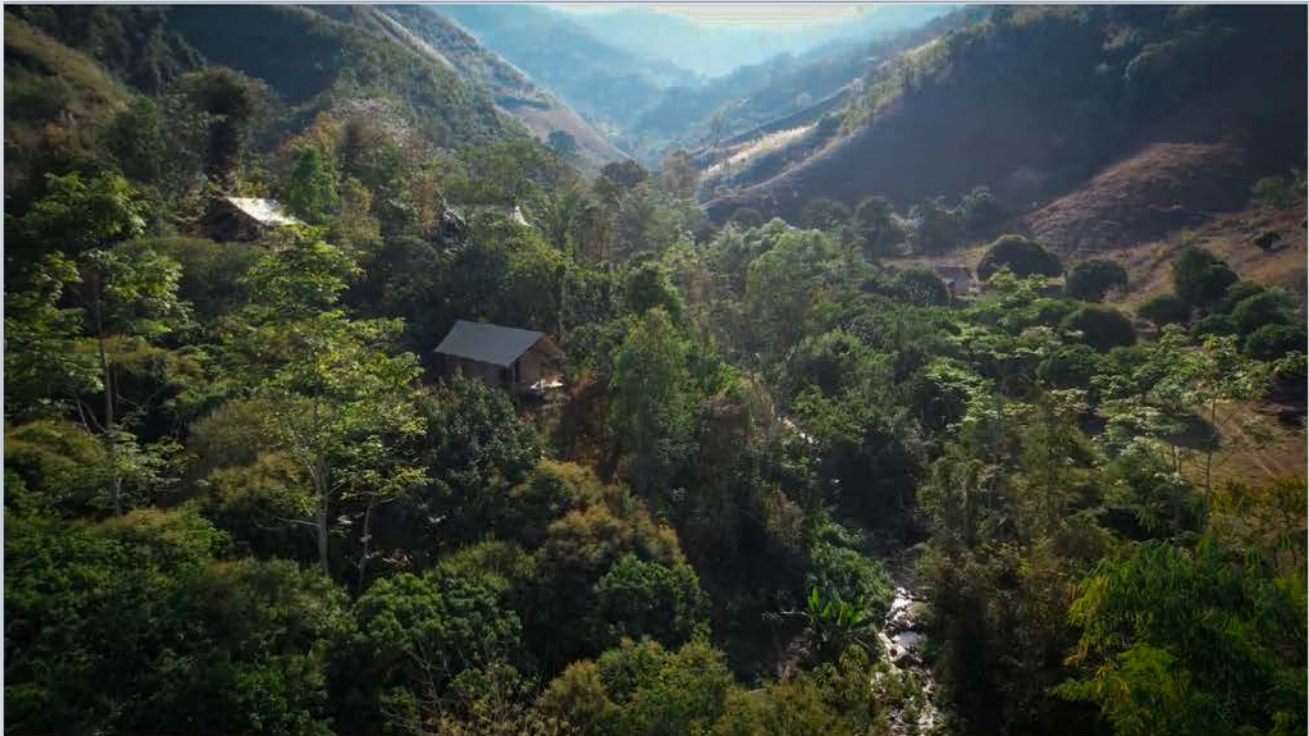
FIGURE 13 Visama by YAANA Ventures — tents threaded into a forested valley and sited along a mountain stream, calibrated to roughly 20 to 24 keys within an hour of a regional airport. Source: YAANA Ventures.
